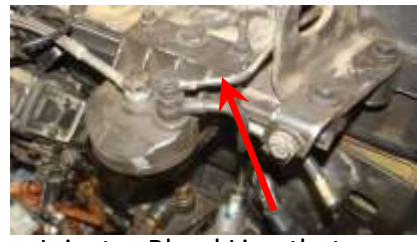
Injector Bleed Line that connects to the tank return line. Figure 55
