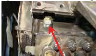
Figure 56 Return Line From the P-7100 Pump
