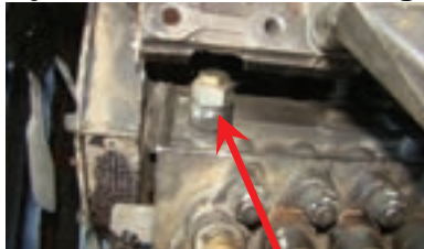
Figure 46 Return Line From the P-7100 Pump
