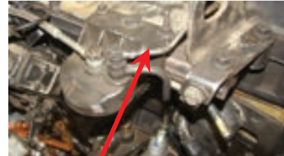
Figure 48 Injector Bleed Line that connects to the tank return line.
